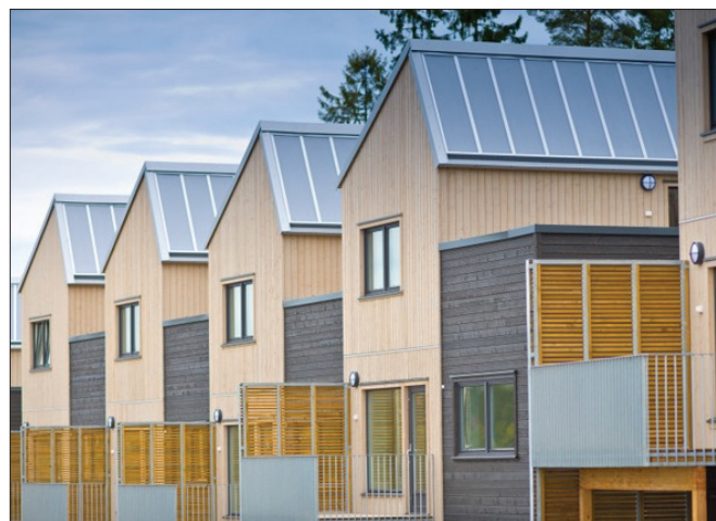
AventaSolar's integrated solar thermal system on residential buildings.
